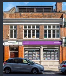
220 Tower Bridge Rd
