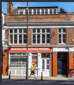
222 Tower Bridge Rd
