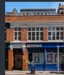
216 Tower Bridge Rd
