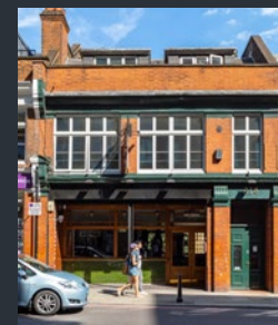
218 Tower Bridge Rd
