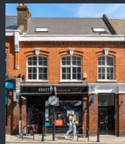
210 Tower Bridge Rd
