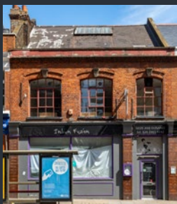
214 Tower Bridge Rd
