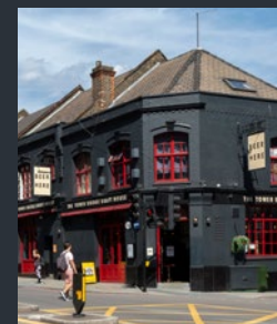
206-208 Tower Bridge Rd
