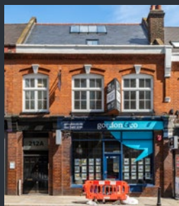
212 Tower Bridge Rd
